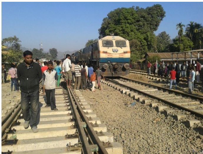
Diesel Engine with ballast hopper rake reached Maibong on 28.12.2014
